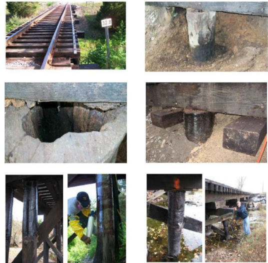
Figure 12. Retrofitting of railroad bridges using FRP wraps, SBVR, Moorefield, WV (July 2010)
