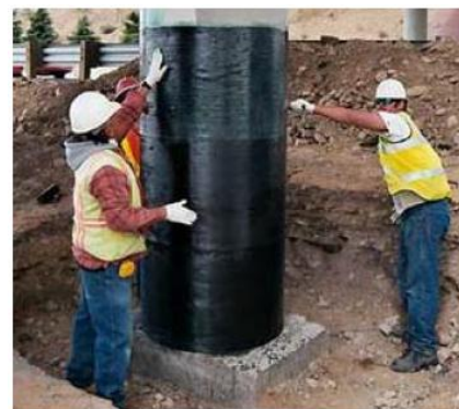
Figure 13. Strengthening of a RC columns with FRPs
