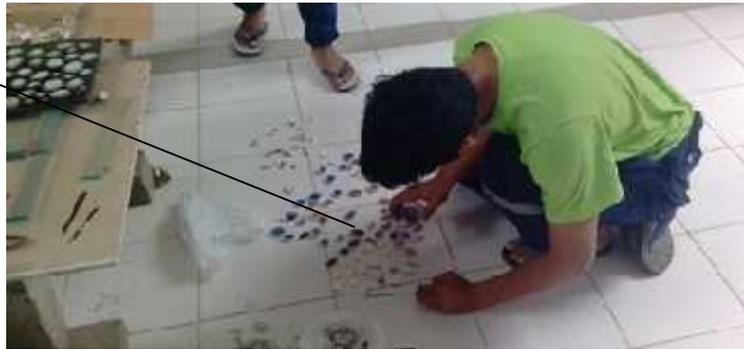
Figure 2. Fan shaped shells filled with a mixture of resin and hardener oils (Source: Author Collections, 2017).
