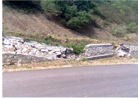
**Gambar 10.** Keruntuhan dinding penahan tanah (Foto dok. Achmad)
