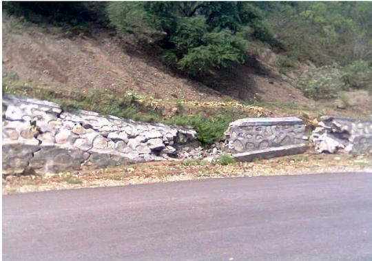
**Gambar 7.** Keruntuhan dinding penahan tanah (Foto dok. Achmad)
