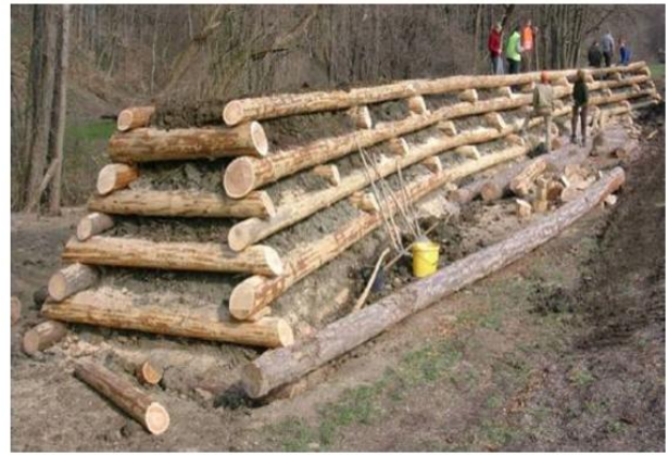
Fig. 2. Wooden log crib wall for noise control in Lower Austria [4]
