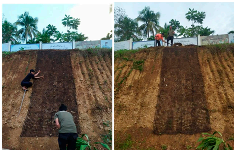
Figure 4. Preparation of embankment and installation of the sugar palm fiber net.
