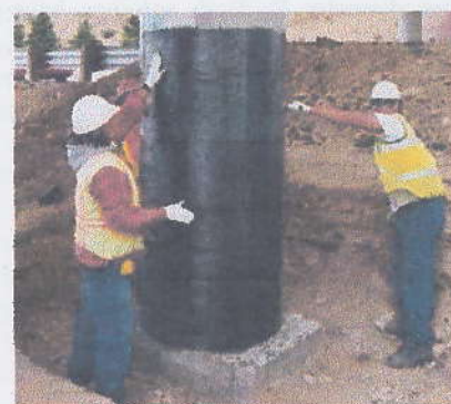
Figure 13. Strengthening of a RC columns with FRPs
