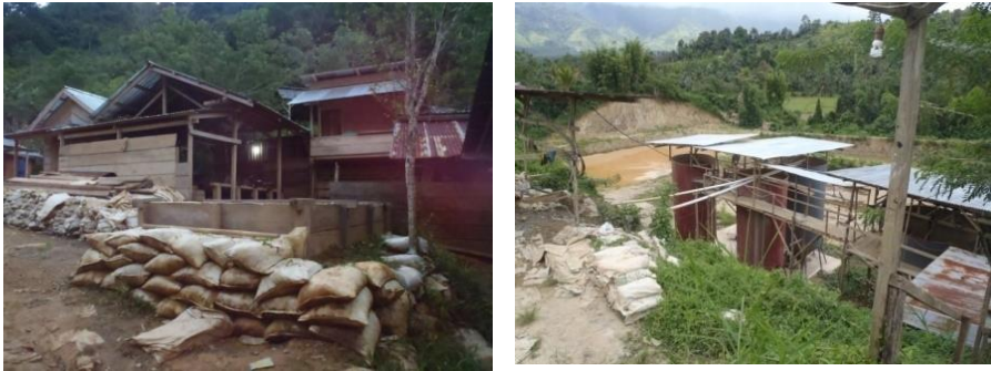
Figure 1. The Tanoyan ASGM site showing Figure 2. The Cyanidation plant in Tobongon, workshop of trommole in back site and bags of three cylinders left and four cylinders right and leftover of sediment waste in the foreground. pond of mining waste is behind.
